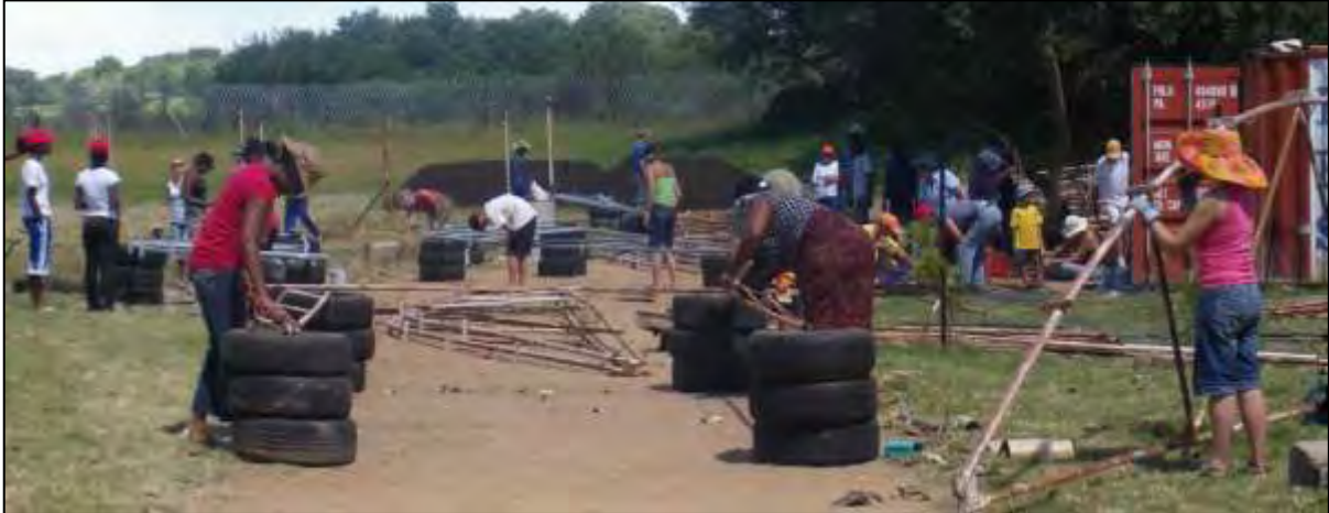
Sand and paint the structure
