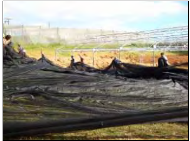
Ready to cover the structure
