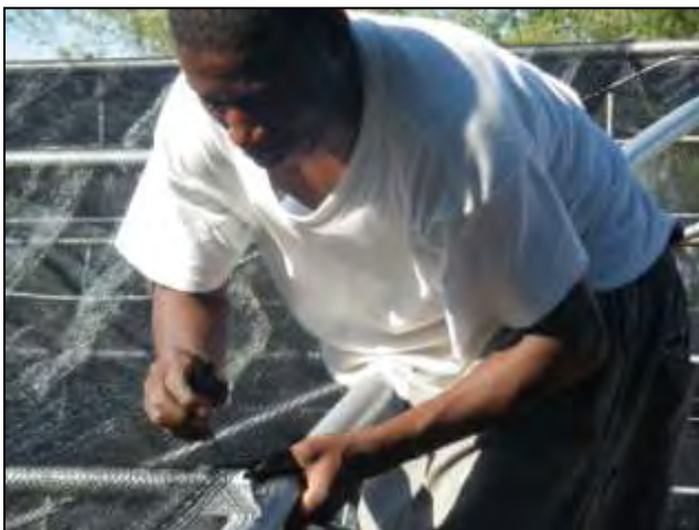
Fix the shade-net to structure
